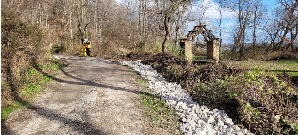
Photo 1 : Downstream of Outlet A looking up the slope showing existing riprap lined drainage channel
