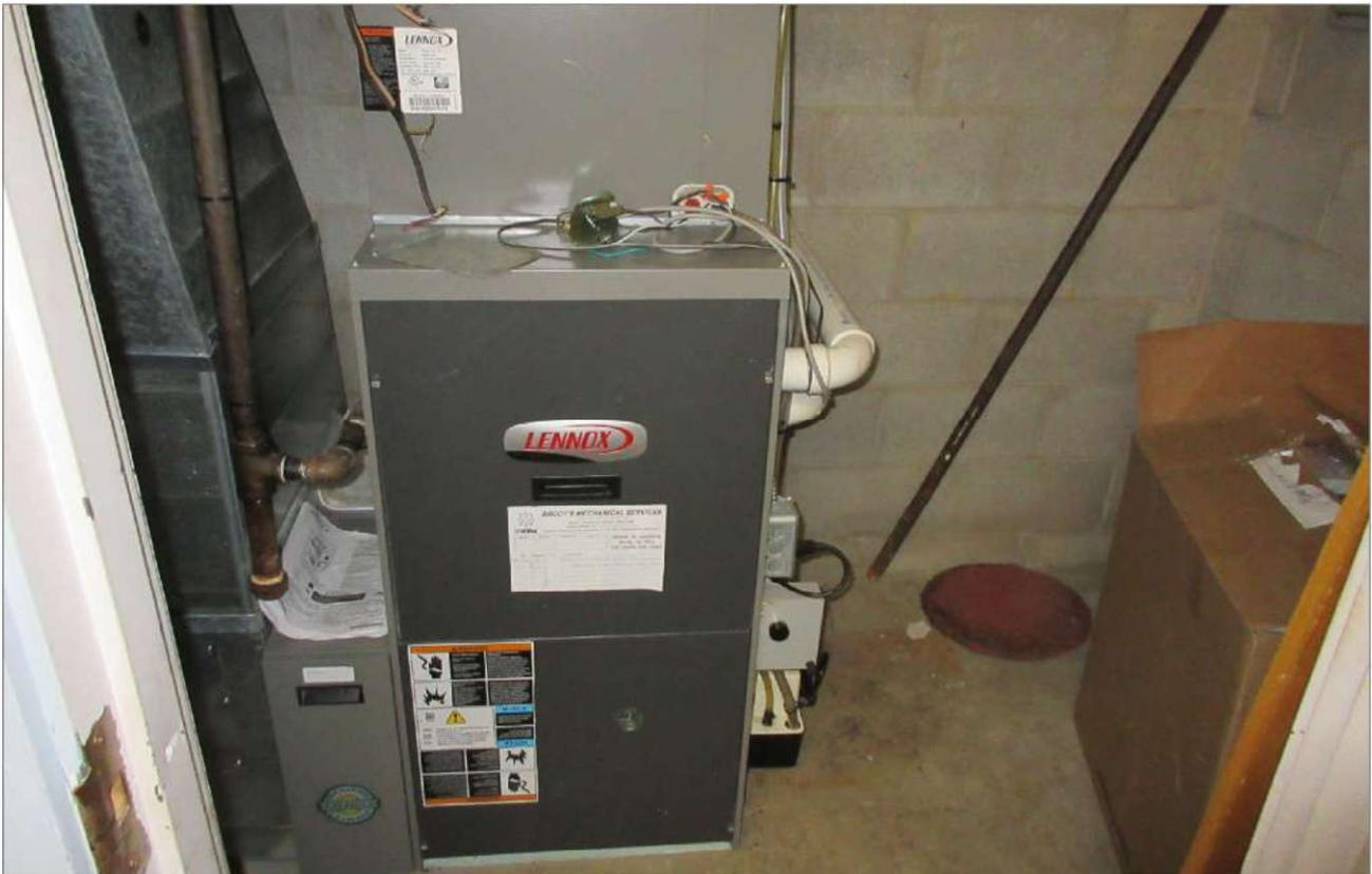
Photograph 22 View of Gas-Fired Forced-Air Furnace at CMHA (Basement)
