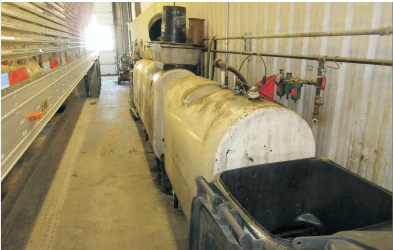
Photograph 34 View of Waste Oil Aboveground Storage Tanks
