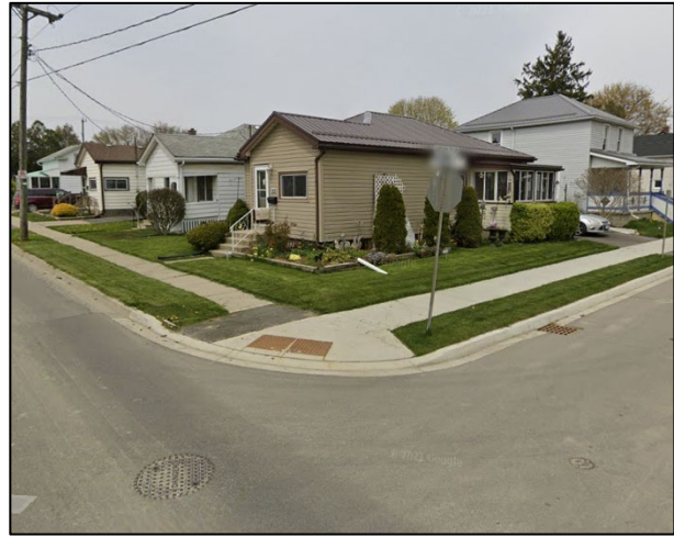
Figure 6 - 149 Stanley Street Exterior Side Yard
