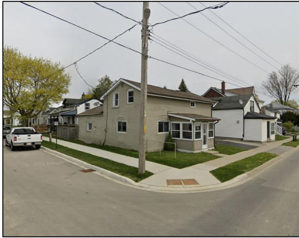
Figure 5 - 145 Stanley Street Exterior Side Yard
