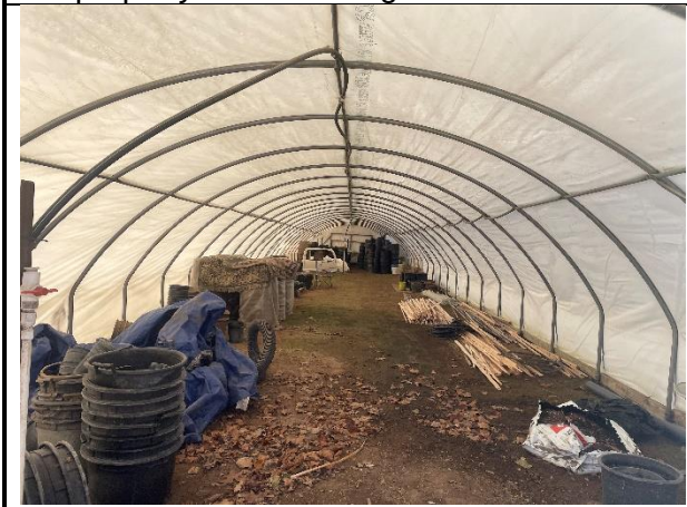
Photo #9: Property 3 – General storage located in the Quonset hut.
