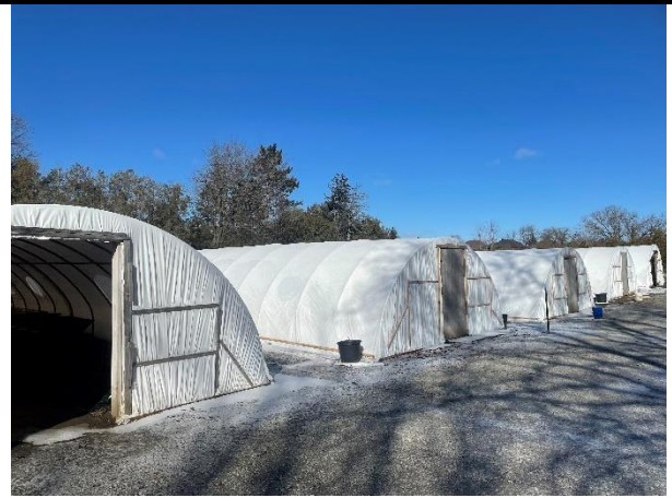
Photo #8: Property 3 – Quonset huts located in the western/central portion of the property.
