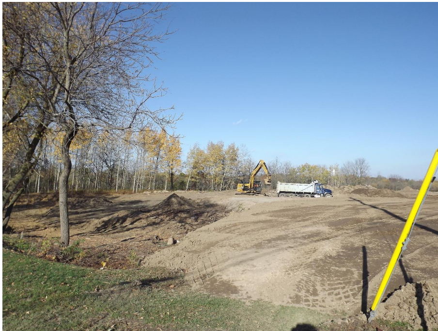
Figure 2: Disturbed project area, facing northeast
